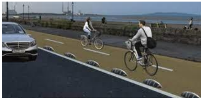
Figure 6-6 Example of a physical bollard between motor traffic and cyclists (image courtesy: IrishCycle.com)
